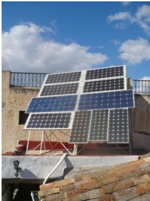
**Image 2.** The photovoltaic solar panels installed on the roof of Sunseed's main property. They supply the vast majority of the electricity used at the house.
