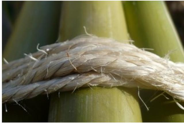
**Image 7.** A column of caña that has been tied together using sisal from the *Agave sisalana* plant.
