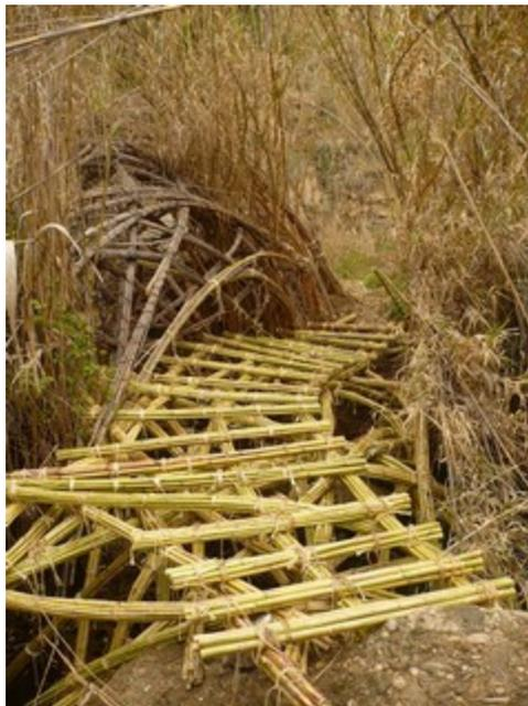
**Image 12.** The cross-struts greatly strengthened the structure of the new bridge.
