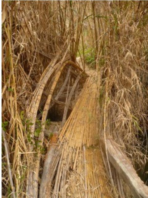
**Image 4.** The old caña bridge. The damage can be seen at the bottom of the photo.
