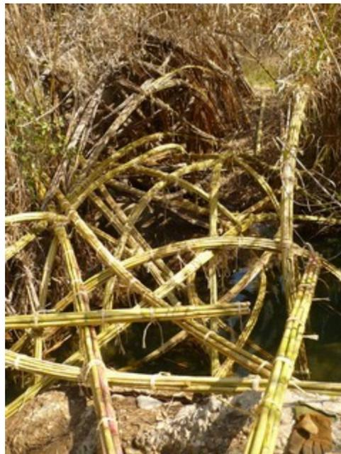
**Image 11.** The foundation structure of the new bridge. The rear of the caña half-dome is just visible in the top left corner of the image.
