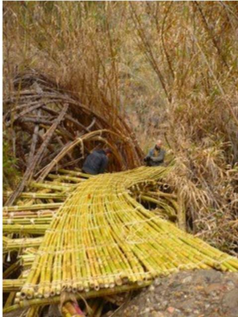
**Image 13.** Tying the walking mat securely to the main structure, bringing the project to an end.
